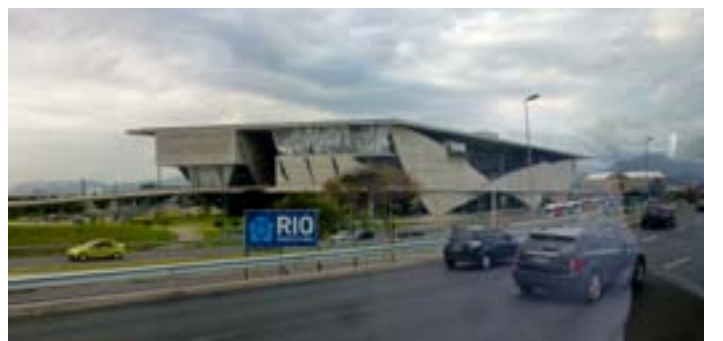
Immediately above: Conference Center, Ciudad des Artes; above, Conservation facility at Museu de Astronomia e Ciências Afins (MAST)
