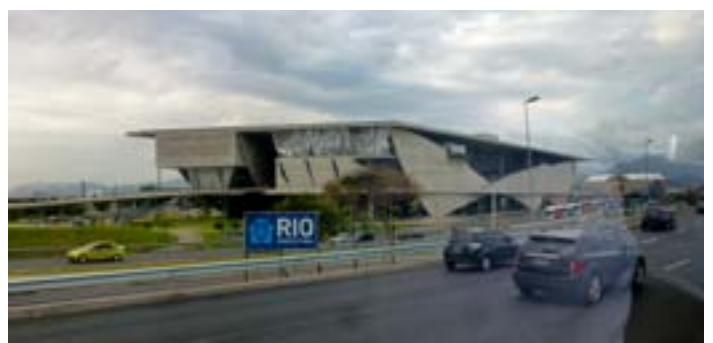
Immediately above: Conference Center, Ciudad des Artes; above, Conservation facility at Museu de Astronomia e Ciências Afins (MAST)
